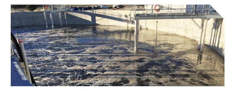
is provided by a cyclic aeration system to create the necessary anoxic and aerobic conditions to promote nitrogen reduction. Phosphorus removal is achieved through a combination of biological and chemical means.
