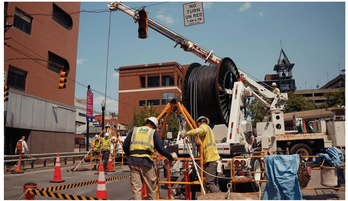
interconnection of the new cable into the existing system. Many circuits branch off multiple times and are comprised of several different cable types, so special attention had to be paid to successfully re-connect into existing cable.
